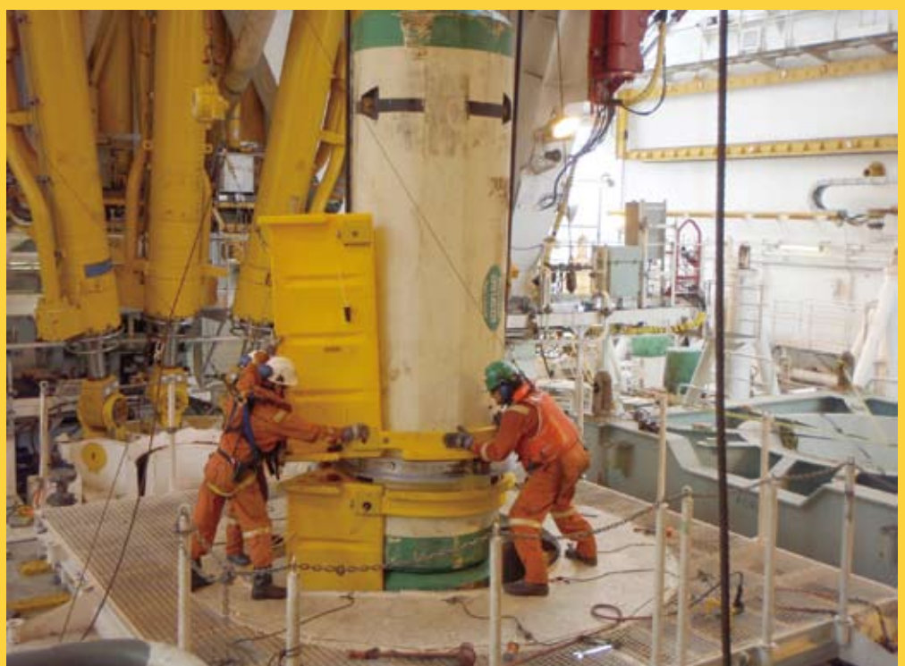
Above: The riser pipe with fairings attached. The picture shows fairing tails pointed in various directions, but they point the same way when placed in an ocean current. Right: Attaching the fairings. One strap is attached using just two pins.
