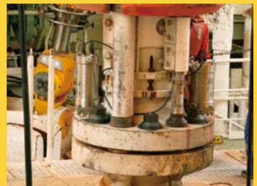
The silver pressure vessels attached to the riser connector are sensors and batteries that record movements.
