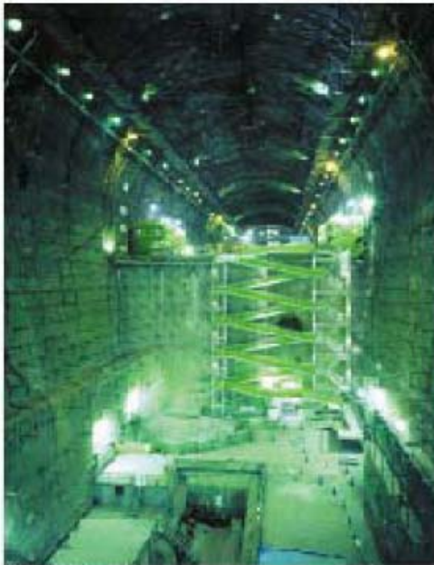
Photo 3: Underground power plant after excavation
