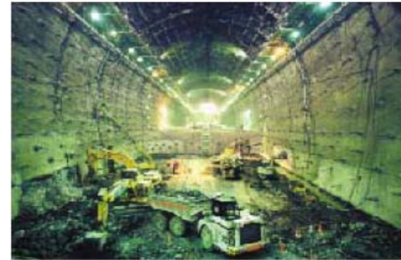
Photo 2: Underground power plant undergoing excavation
