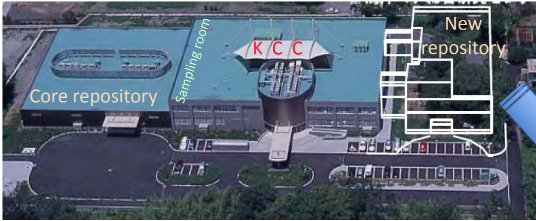
Aerial view of KCC
