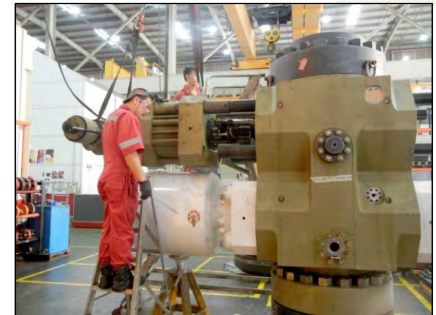
Double body (Cameron) Replaced with new ones - SSR
