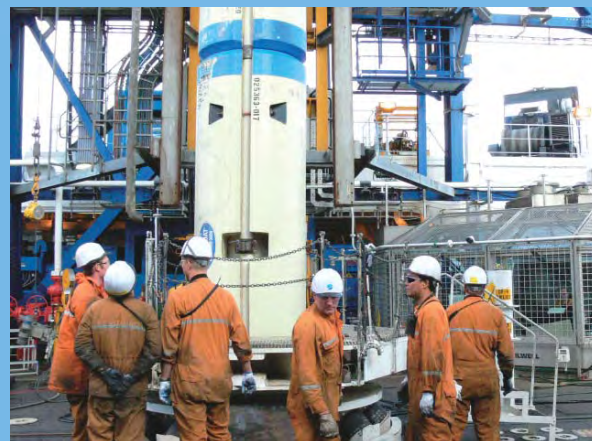
On the drill floor while assembling the riser pipe
