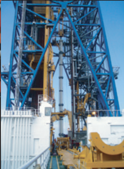
A riser pipe set vertically in the derrick. It is lowered to the ocean floor from the moon pool.
