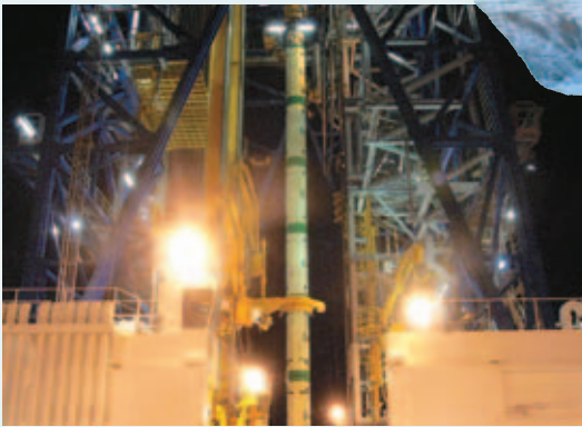
Lowering the riser pipe (center) into the sea. Chikyu has already successfully drilled to more than 3,000 meters below the seafloor with riser drilling during the shakedown cruise.
