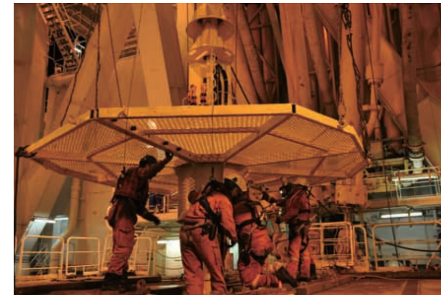
The ROV platform and the top of the Long-Term Borehole Monitoring System observatory being connected together. These sections sit on top of the wellhead at the sea floor. The diameter of the platform is approximately 5 m.
