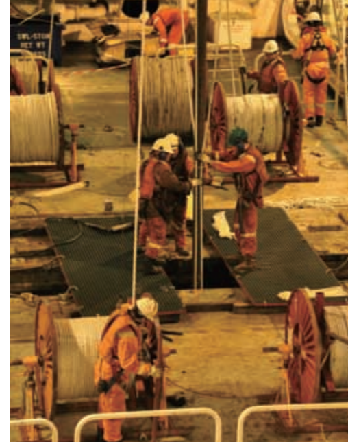
Vibrations caused by the Kuroshio Current can be suppressed by attaching 4 lengths of rope along the drill pipe.
