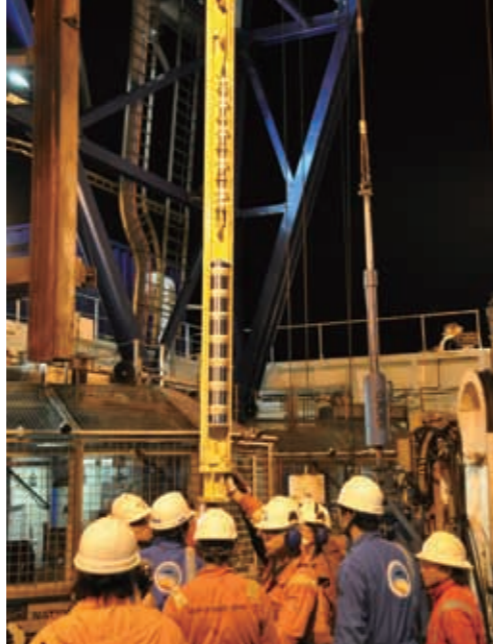
With the instrument package attached, the assembly of the almost 7 m frame is finished (in front).
