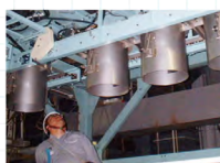
Big Bag Filling System Fill stabilized sludge in big bag
