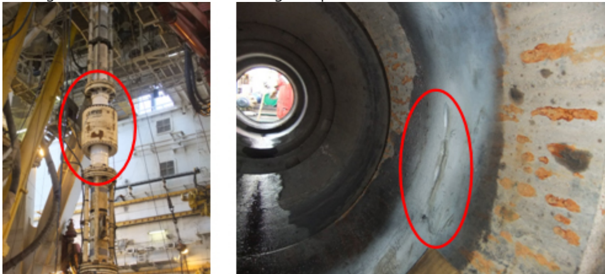
Figure 1 Damaged equipment (left) and cracks inside the equipment (right).
