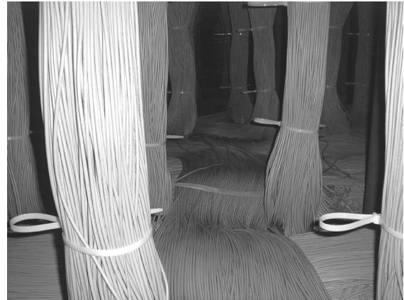
Photo 14 Internode cable in free access floor.
