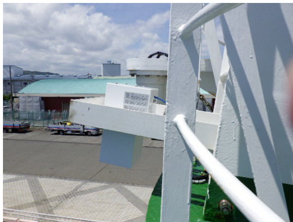
Figure 3.6-1 Microwave wave gauge installed at the bow.
